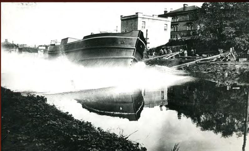
J. & J. Hay, S.S. 'Serb', built in 1927. Hay's built over 60 puffers. They were launched sideways into the canal
