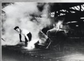
Moulders pouring molten iron from ladle into moulding box, 1950s (The Scotsman)
