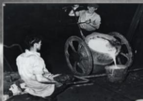
Moulder pouring molten iron from bogie into a ladle, 1950s
