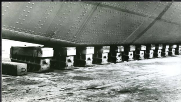
Keel blocks under liner. These heavy duty cast iron blocks were used to support the weight of large ships.
