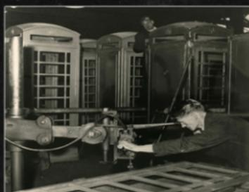
Worker drilling a panel of a K6 telephone kiosk in the finishing shop of the foundry, 1950s
